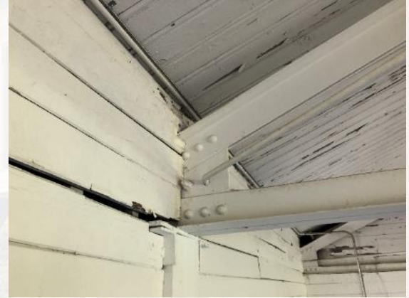
Settlement at Top of Column
