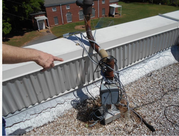
Abandoned Services on Flat Roof
