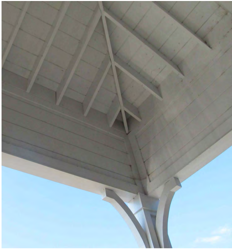
FIG. 4: EXISTING WOOD ROOF. NEW WORK TO REPLICATE ROOF STRUCTURE.
