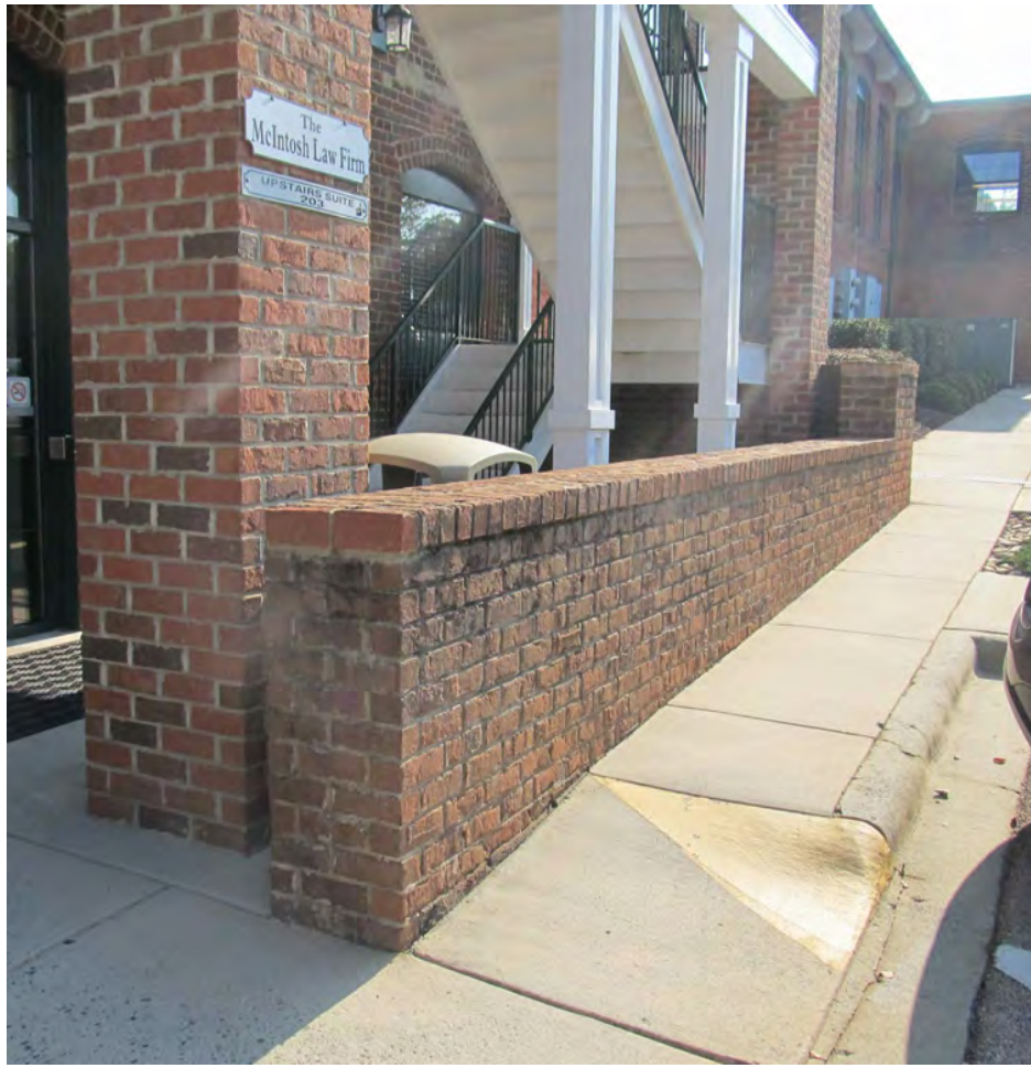
FIG. 5: EXISTING SIDEWALK IS VERY STEEP AND NARROW. NEW SIDEWALK WILL WIDEN THE WALK AND ALLOW THE SLOPE TO BECOME MORE SHALLOW.
