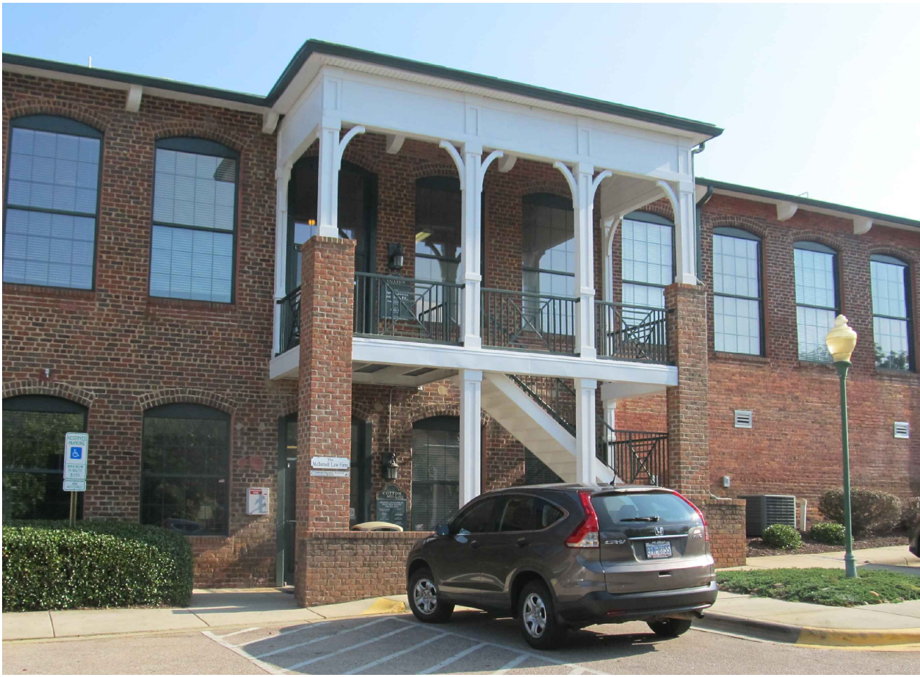
FIG. 2: EXISTING BUILT FORM CONTAINING METAL-PAN STAIRS AND SECOND-FLOOR PLATFORM.
