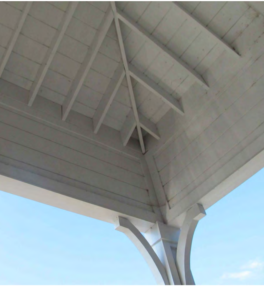
FIG. 4: EXISTING WOOD ROOF. NEW WORK TO REPLICATE ROOF STRUCTURE.
