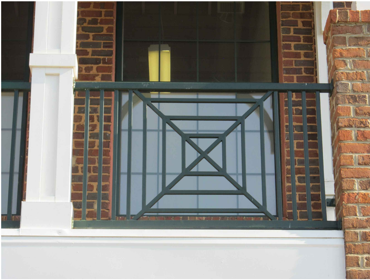
FIG. 3: EXISTING GUARDRAIL MOTIF TO BE MAINTAINED IN NEW WORK.
