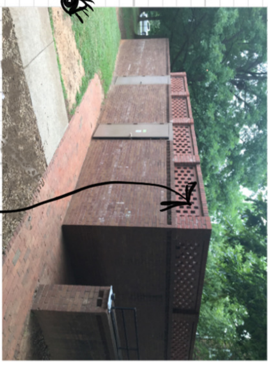
EXISTING MASONRY WALL w/ RAINING 16\"/>
