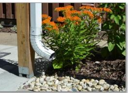
**Vegetated Swale** Shallow ditch with plant cover; natural infiltration.
