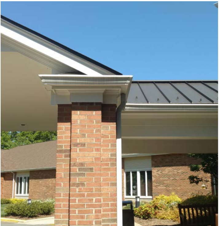
STANDING SEAM METAL ROOF AND BRICK COLUMN
