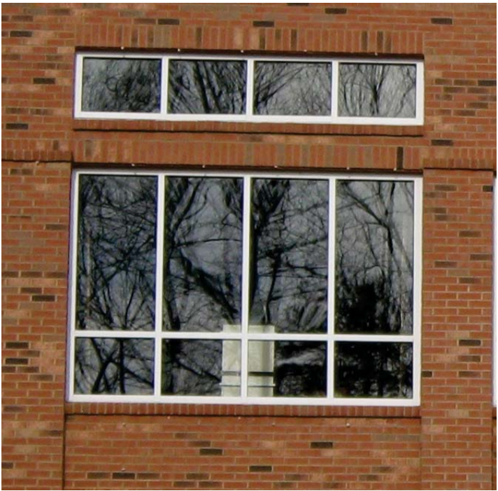
SOILDER COURSE AND BRICK LEDGER DETAILS
