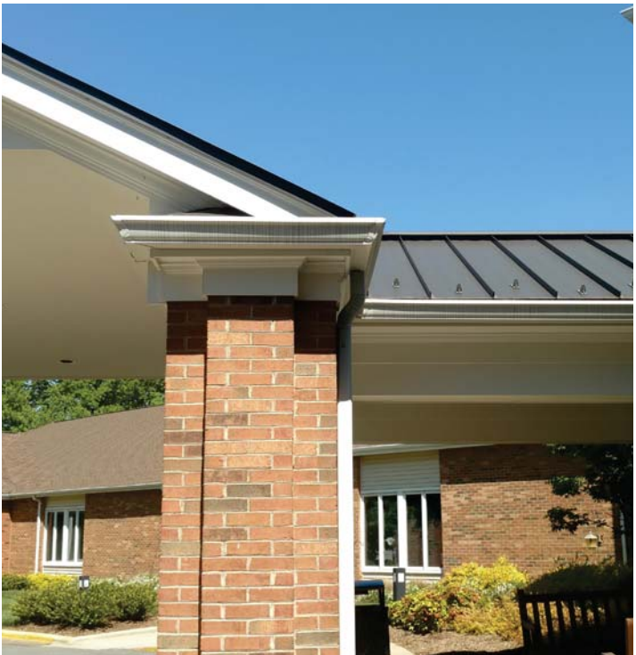
STANDING SEAM METAL ROOF AND BRICK COLUMN
