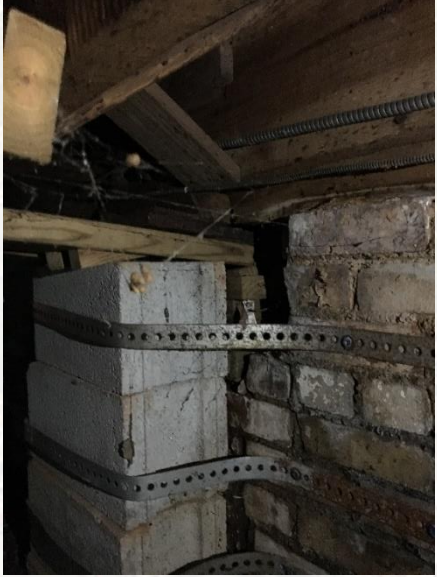
Foundation Repair Front Wall
