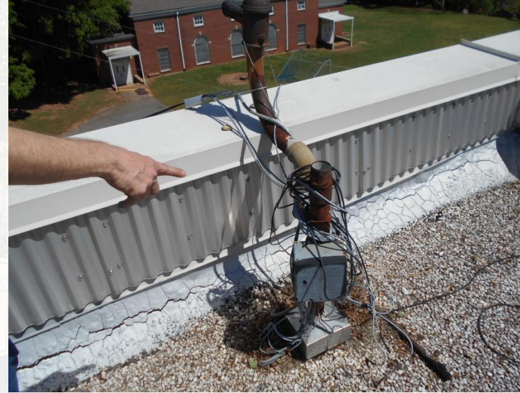
Abandoned Services on Flat Roof
