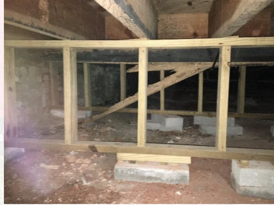
Floor Structure Repair
